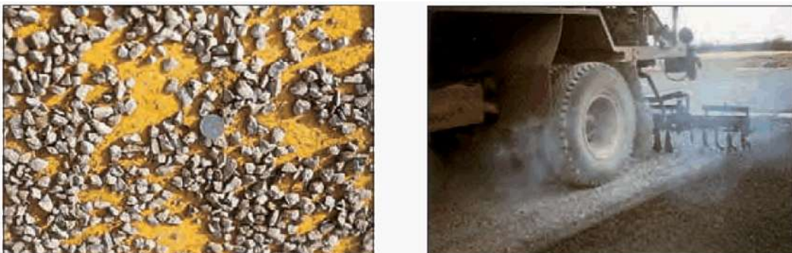
Figure 25 : Protection superficielle (source SETRA)
