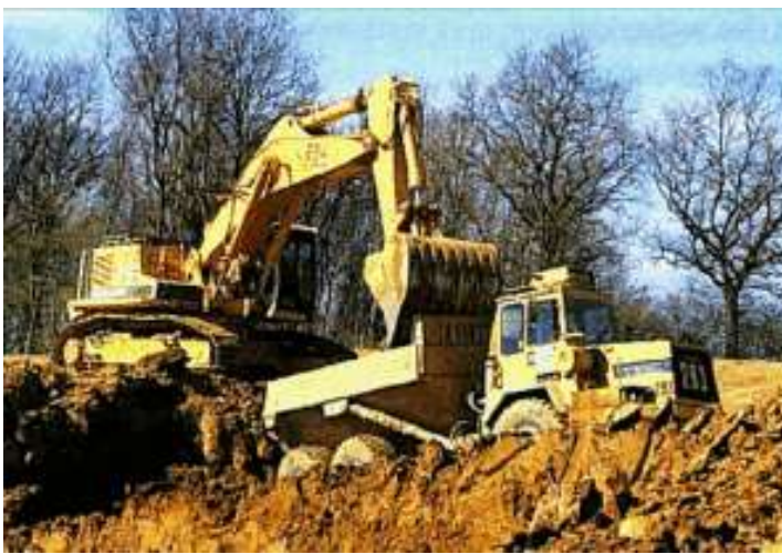
Figure 12 : Extraction frontale (source : SETRA)
