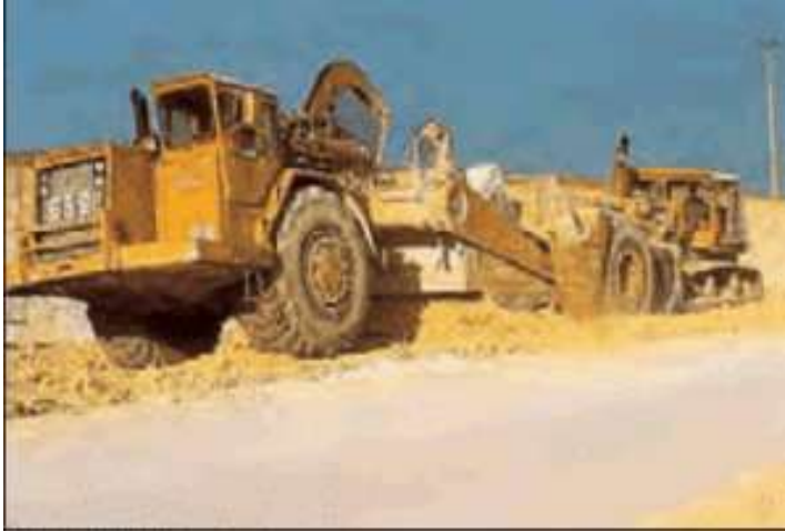
Figure 11 : Extraction frontale (source : SETRA)
